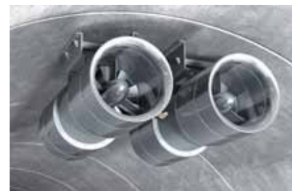
Ventilatori in tunnel
